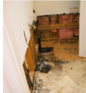
Mold Remediation Bathroom
